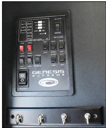
Central Monitor/Control Panel
