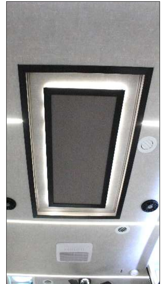
New Design Ceiling Soffit Lighting
