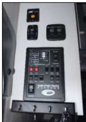
Convenient Monitor & Lighting Control Center
