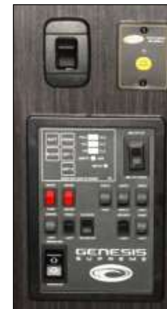
Centralized Monitor, Lighting & Inverter Controls
