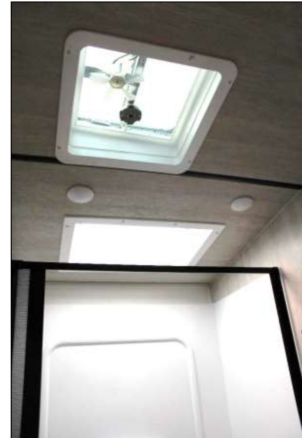
12-Volt Powered Lavy Vent Fan & Skylight Above Shower
