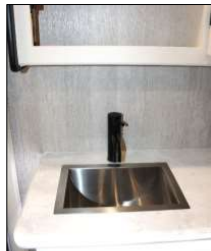
Metal Lavy Sink w/Single Handle Fixture / Mirrored Medicine Cabinet
