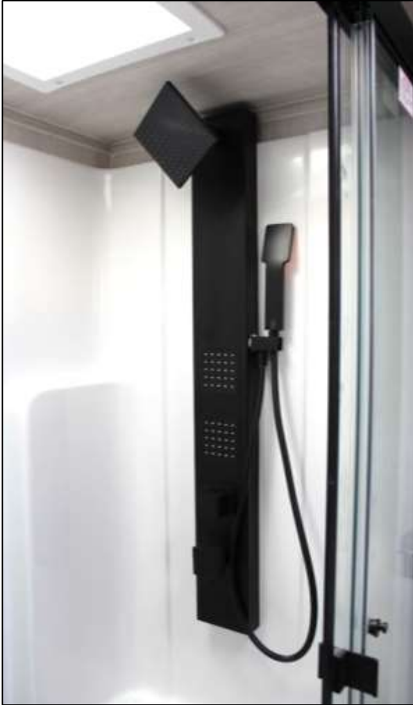
Large Shower with Designer Fixtures & Skylight Above
