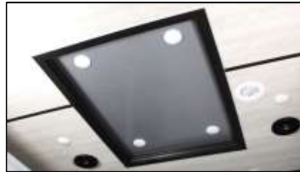
Decorative & Functional Overhead Lighting
