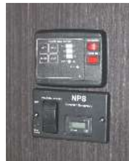
Convenient Water Pump/Water Heater Controls
