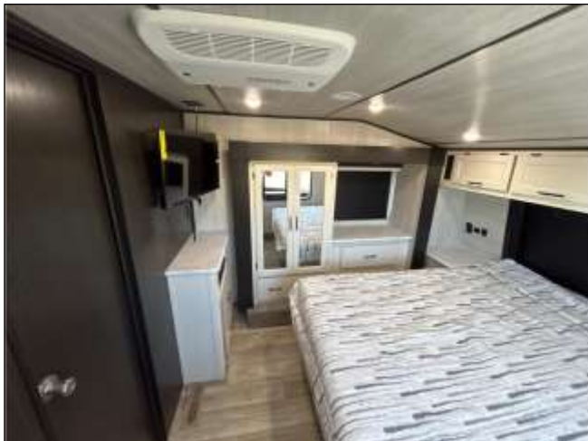
Ceiling-mounted A/C with wall-mounted Controls
