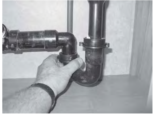
Typical galley/bath P-trap and drain fittings
